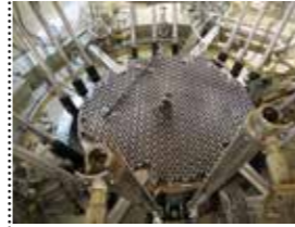
© Nucleoelectrica Argentina S.A.
